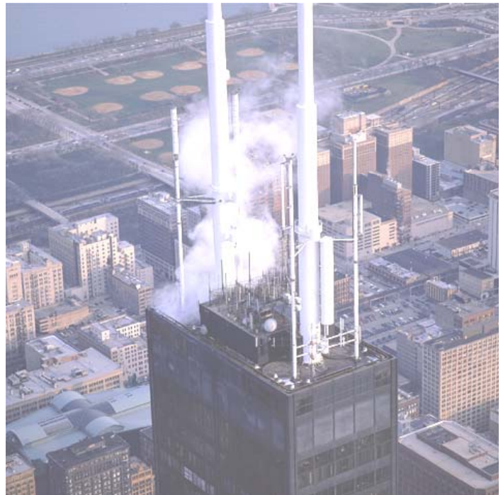
Figure 1: Panel and Slotted Coax Arrays on the Sears Tower, Chicago, IL
